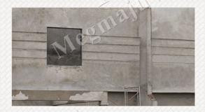
Allow one week for the smooth outer layer to cure before painting the wall to the desired colour. The reason why a week curing is necessary is to make sure that all the plastered walls are free from hairline or large cracks in the plaster before proceeding on the final touch which is painting.
