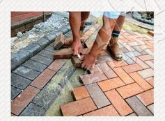
**8. Cutting in the edges** Mark the blocks before cutting.
