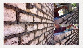
The right way to apply plaster is to apply a thin coat of mortar (1:3) on the inner wall and followed by a thin coat (1:4) of mortar on the outer wall while waiting for the first inner coat to dry. Repeat by alternating between the inner and outer wall until the desired thickness of plaster is achieved. The thickness of the plaster should cover up the wire
