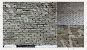
Bricks already install should sprinkle or pour water from top to bottom to separate and make it water-proof. Usually pour water for consecutive three days before plastering.
