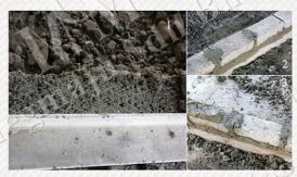
Made of Steel Reinforce Rods- Four Steel Wire Rod (size depends on plan) form to square type (length as per plan) for every one feet at pole side attached (tying) Brick Wire Mesh at the Steel Rod, for trying use Galvanized GI Wire. After settled all the Brick Wire Mesh up to the end line of the pole (each side of the pole covered with any used wood) then pour the mixed concrete.
