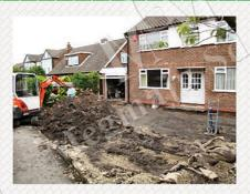
**2. Excavation**Dig as required & dispose excess soil.
