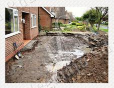
3. **Sub-base**Spread the sub-base to have flat even surface.
